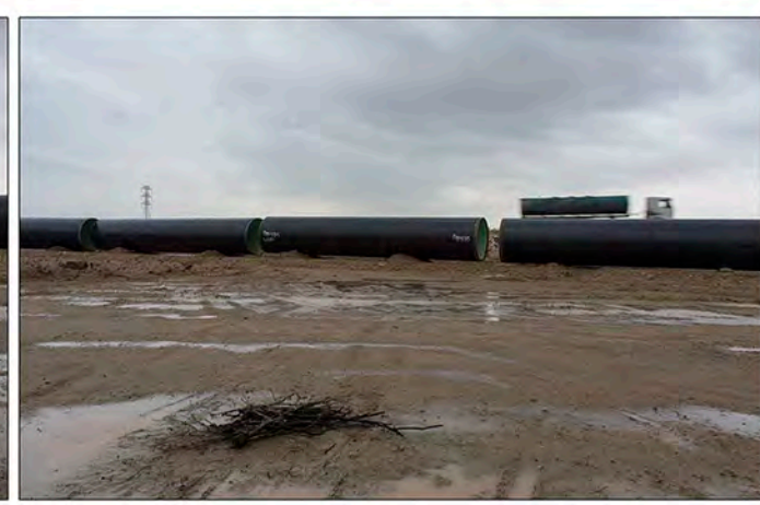
Installation of Steel Pipeline 2000 mm Diameter
