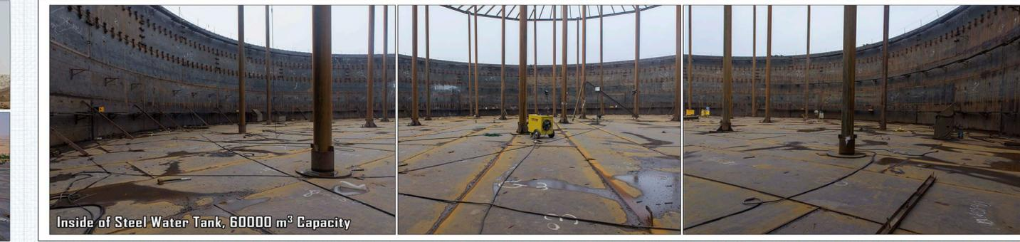
Inside of Steel Water Tank, 60000 m<sup>3</sup> Capacity
