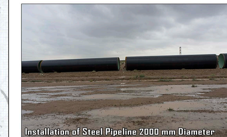
Installation of Steel Pipeline 2000 mm Diameter
