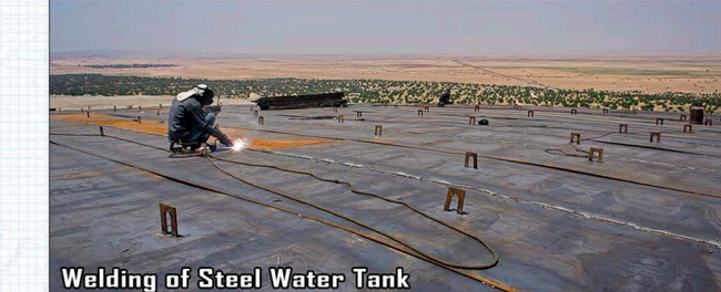
Welding of Steel Water Tank
