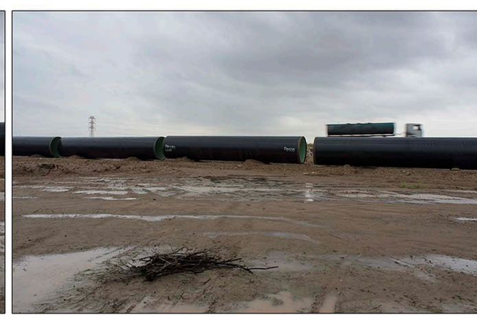
Installation of Steel Pipeline 2000 mm Diameter
