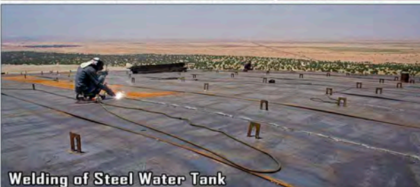
Welding of Steel Water Tank
