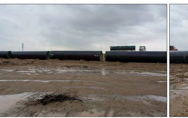
Installation of Steel Pipeline 2000 mm Diameter
