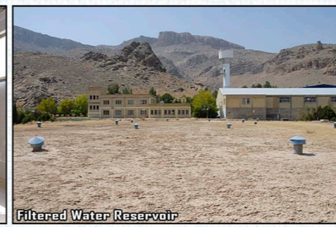
Filtered Water Reservoir
