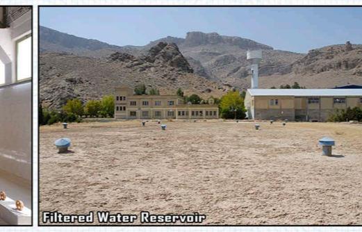
Filtered Water Reservoir
